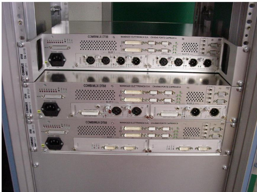
2. Connectors accessible from the front with equipment placed backwards to avoid connectors from protruding
